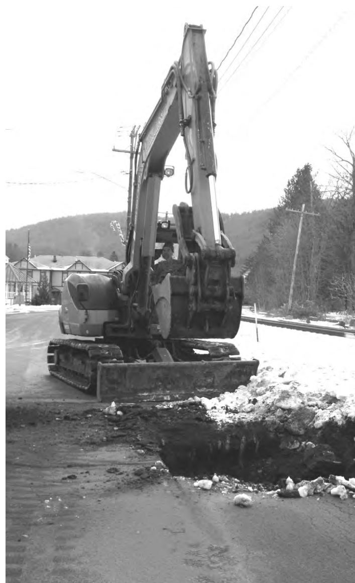
The Village of Hancock crew, along with some Town of Hancock employees, performed "exploratory surgery" at the intersection of Front Street and Wheeler Street on December 26, looking for a leak in the water main.
